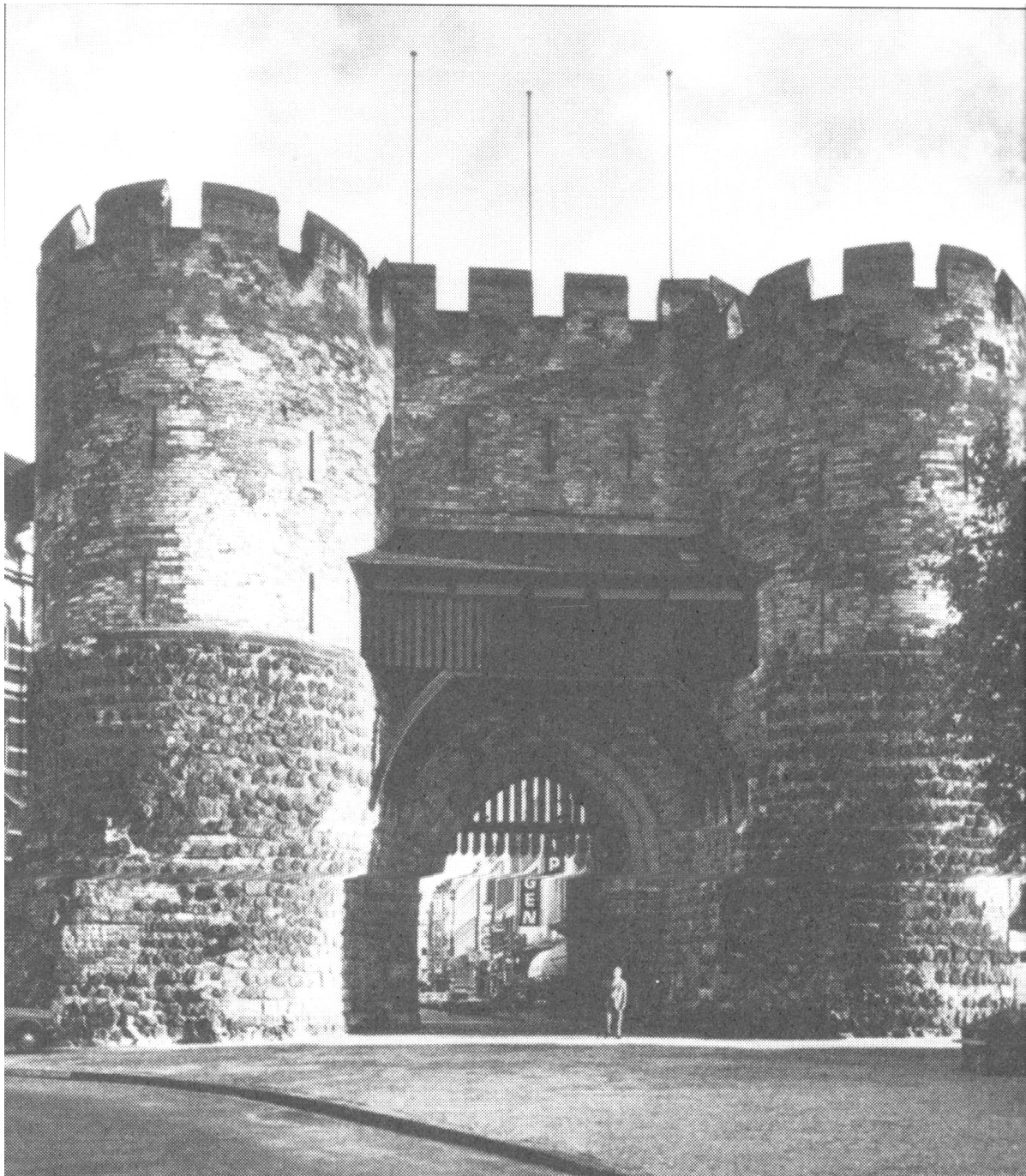
Figure 4: Cologne, Eigelsteintor, from: Biller, Stadtmauern , 100
