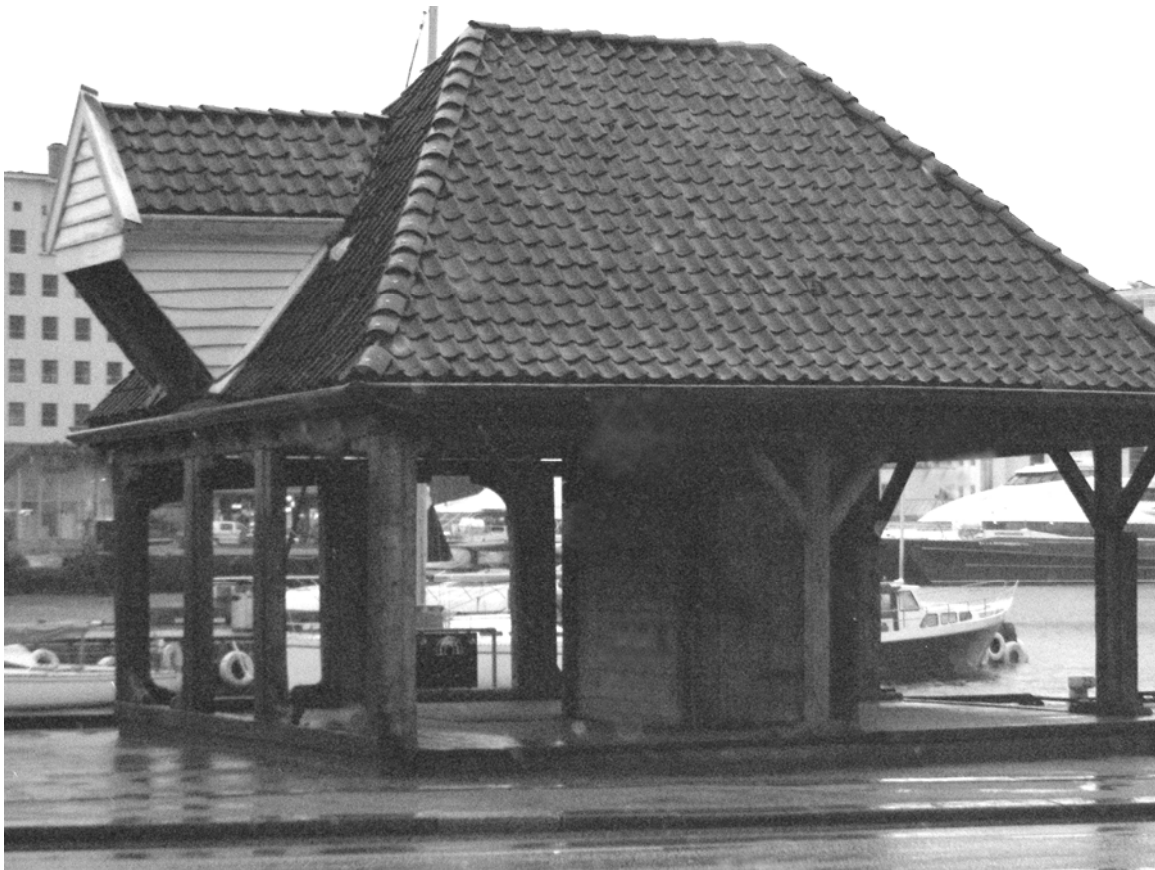
Figure 2: The reconstructed public latrine house in the Bryggen district of Bergen
