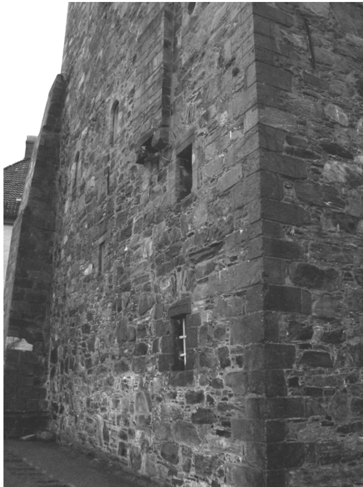
Fig. 1: The remains of the overhanging latrine on Rosenkrantz Tower in Bergen are still visible
